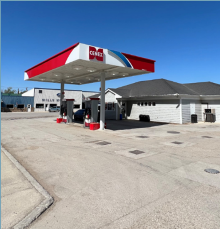
Our Fairfield team emptied everything out of the old store and moved the inventory to our farm store to prepare for the demolition.
