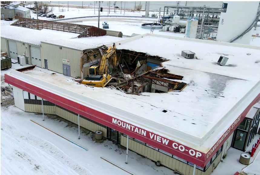
Excavators started demolishing the old building on March 8th, 2022.
